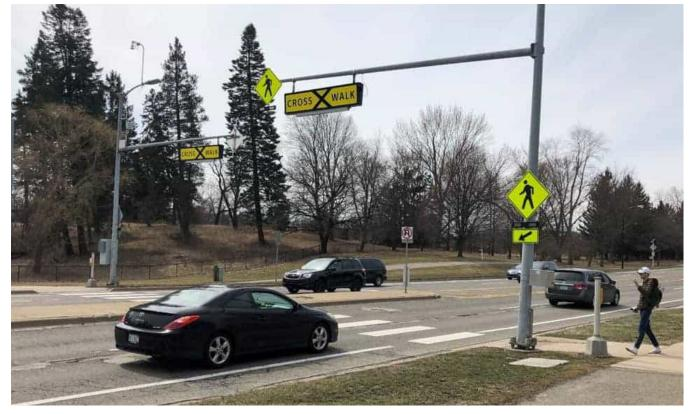
Recangular Rapid Flashing Beacon and pedestrian crosswalks support the safety of pedestrians at crossings
