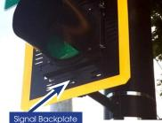
Signal backplate framed with a retroreflective border. Source: FHWA
